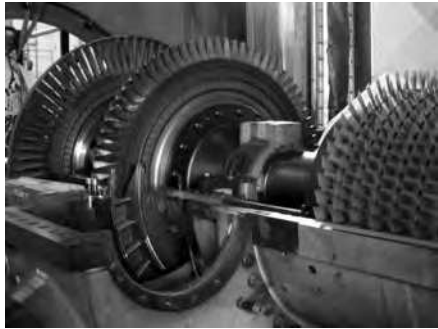
(a) Example of a gas turbine. (Source: OGE.)
