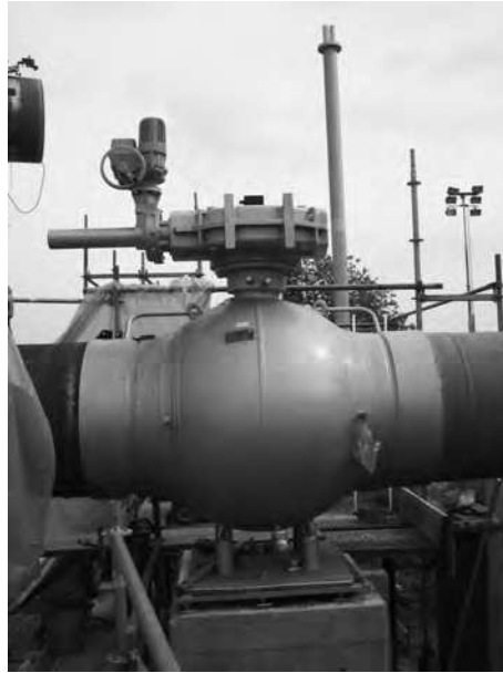
Figure 2.2. A ball valve. (Source: OGE.)
