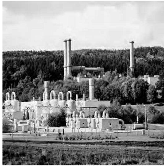
Figure 2.9. The compressor station in Waidhaus, Germany. (Source: OGE.)
